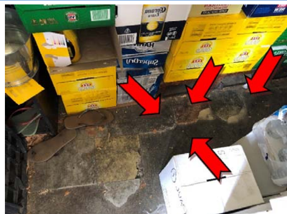
Photo 12. Interior, storage area behind bar, floor coverings (red, yellow, black & blue) – asbestos-containing vinyl floor tiles and adhesive.
