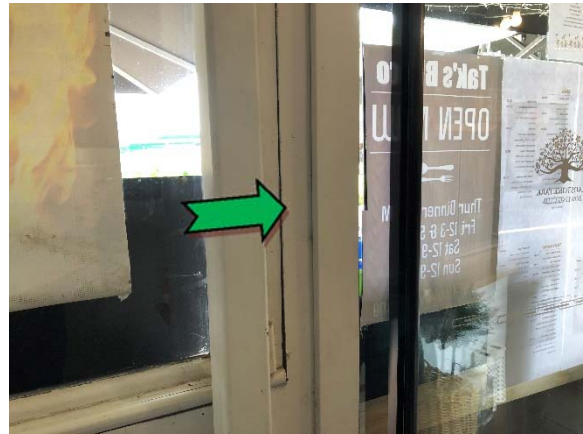
Photo 16. Interior, adjacent gaming room, corridor, infill panel – non asbestos-containing fibre cement sheeting.
