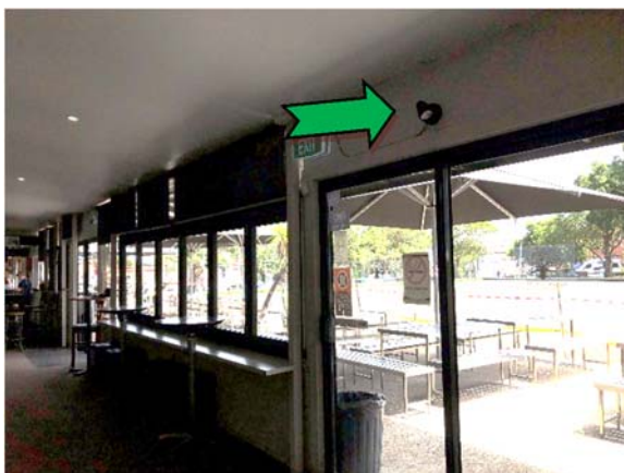
Photo 17. Interior, north-west elevation, door position, infill panels – non asbestos-containing fibre cement sheeting.
