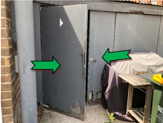
Photo 1. Exterior, shed, external walls and door – non asbestos-containing fibre cement sheeting.
