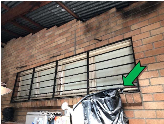
Photo 21. Interior, north elevation, garage/store, window frames – non asbestos-containing window caulking.
