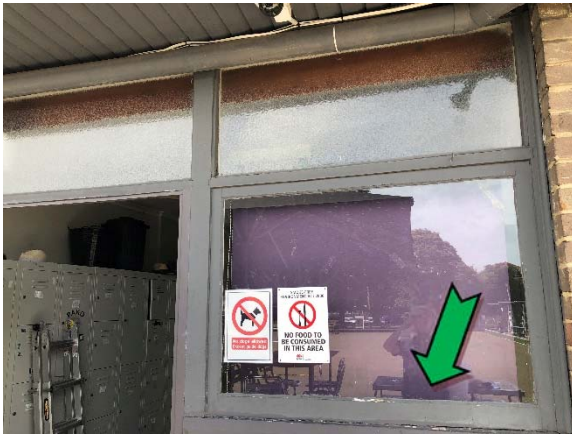
Photo 3. Exterior, locker room, window frames – non asbestos-containing window caulking.
