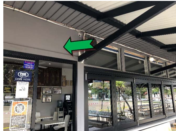
Photo 4. Exterior, north elevation, wall – non asbestos-containing fibre cement sheeting.
